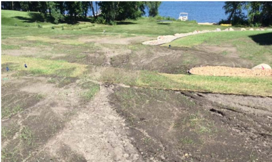
Left: Erosion caused by not having proper vegetation growth >80% prior to removing the silt fence between the slope and Sauk Lake.
