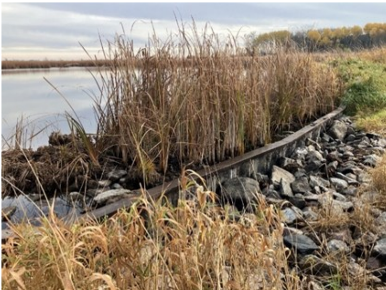
Krantz Lake weir, fall 2025
