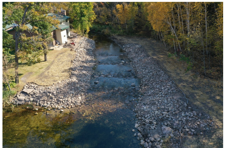
Completed rock arch rapids at outlet of Little Birch Lake near Grey Eagle, an SRWD project
